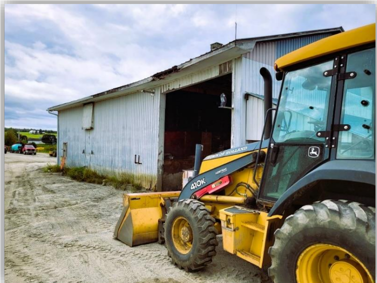
Town Garage Back, Photo Credit - Stacy Boone
