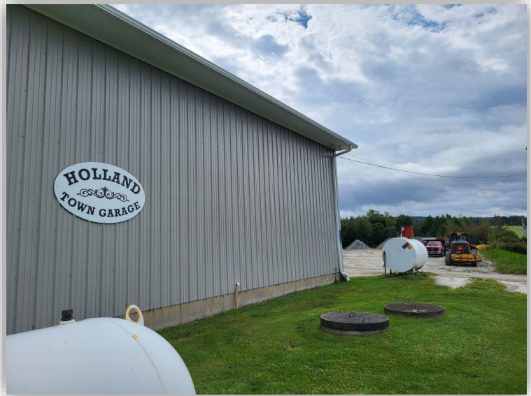
Town Garage Road View, Photo Credit - Stacy Boone
